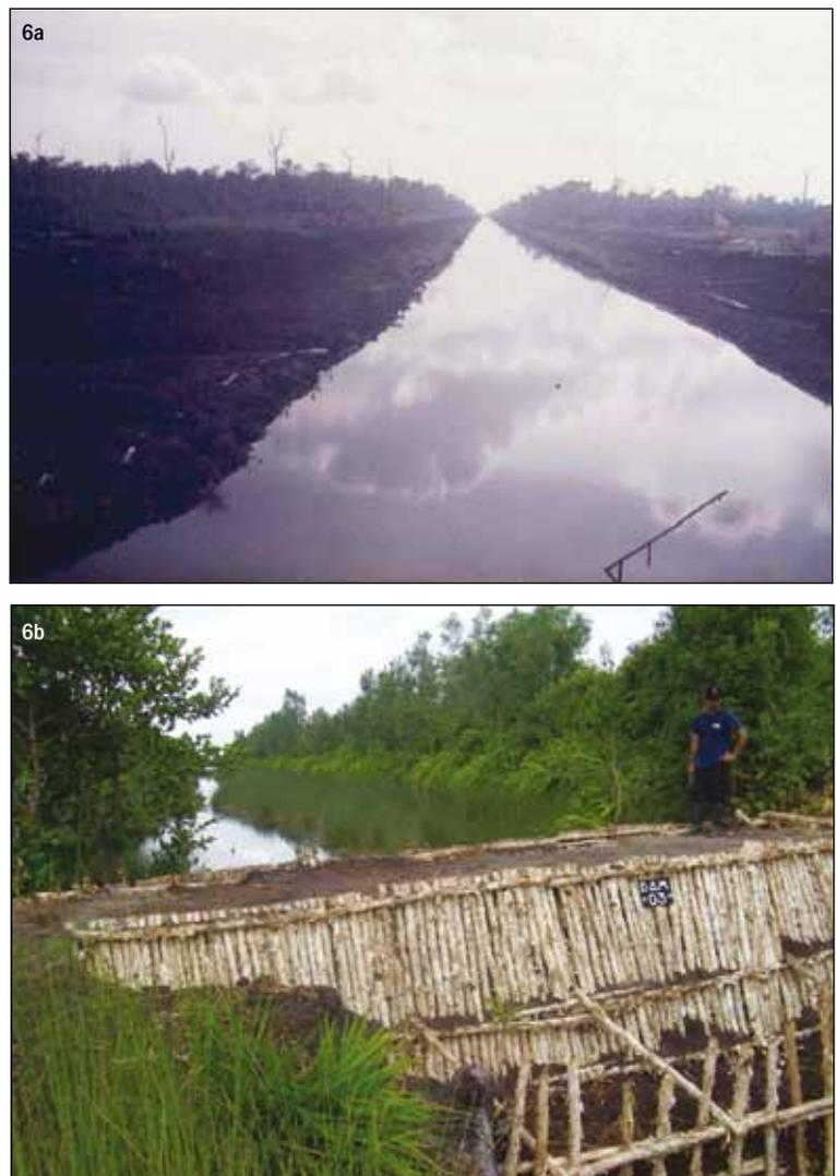
**Figure 6.** Large drainage canal in the ex-Mega Rice Project area when first dug in 1997 (a) and after (b) damming. Note the width of the canals and the difference in water level above and below the dam in Figure 6b. Photographs by CIMTROP.
